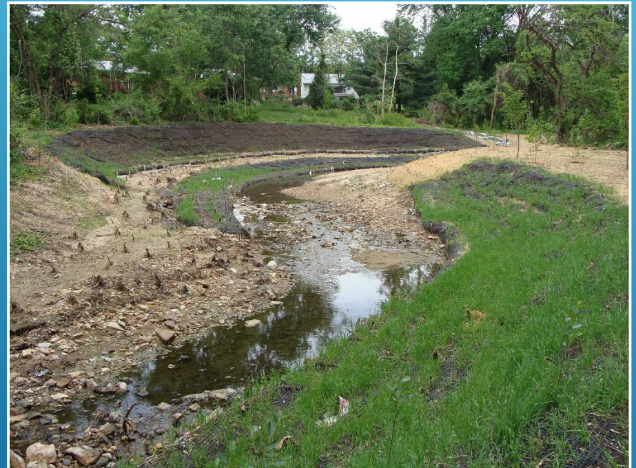
Soil lifts and vegetated banks soon after construction
