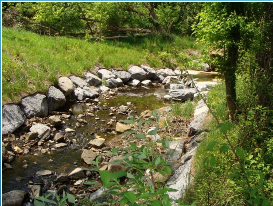
Rock toe protection soon after construction
