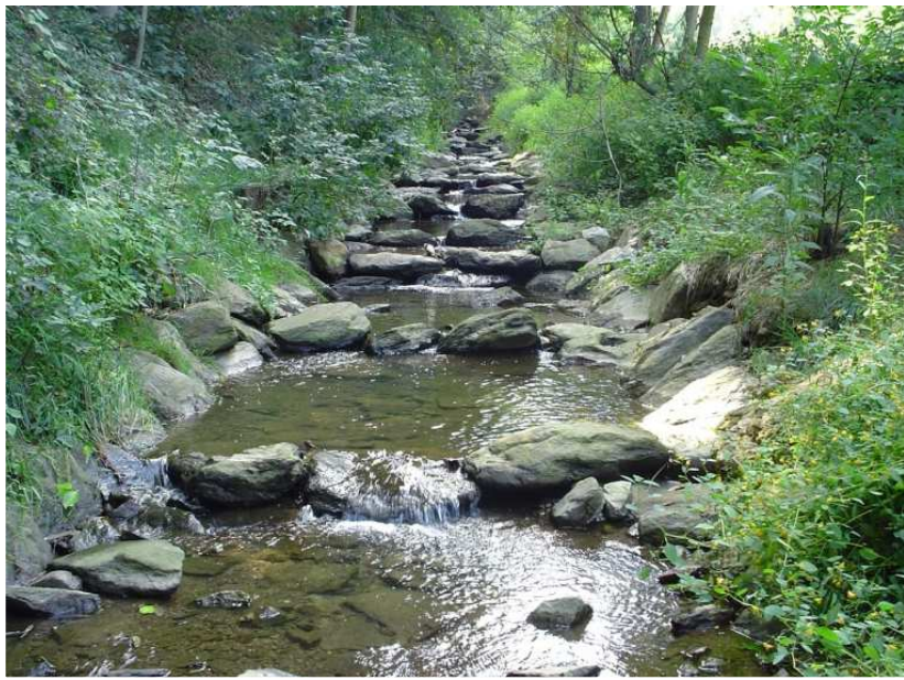
Step pools expend energy vertically – Goodwin Run, completed 2001
